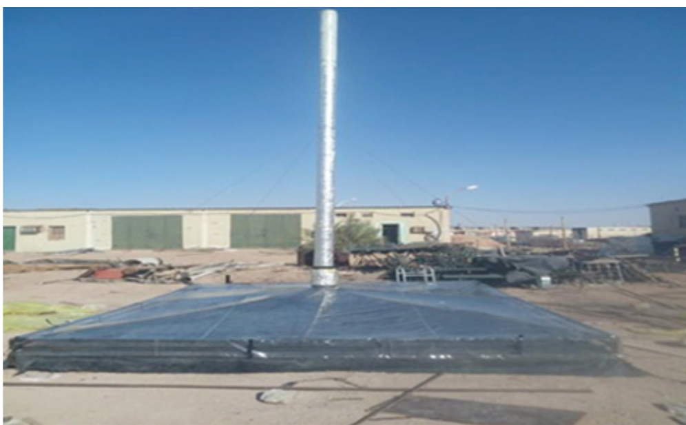
Fig. 1. Photo of the small scale solar chimney in Ouargla.
