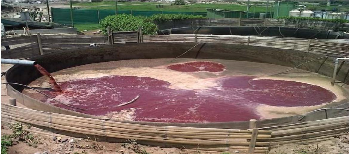
Fig. 1. Storage of the meat effluent in the equalizing tank after pretreatment (screening and sedimentation).
