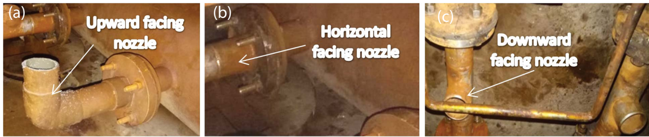
Fig. 2. (a) Upward nozzle, (b) horizontal nozzle, and (c) downward nozzle.
