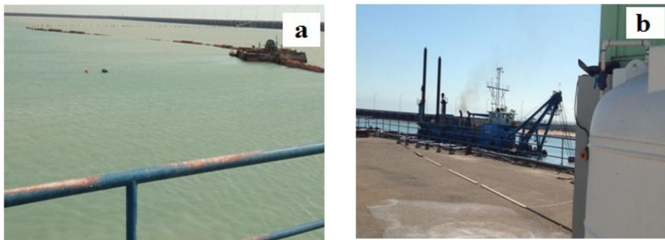
Fig. 1. (a) Turbid seawater at SDPI's site and (b) dredging of the seawater intake inside the Sabiya Power Generation and Water Desalination Plant.
