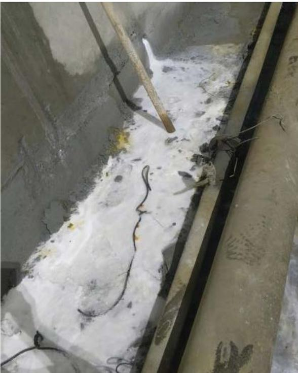
Fig. 1. Drainage pipe blocked by crystals in the Baoligang Tunnel along the Emei-Hanyuan Expressway.
