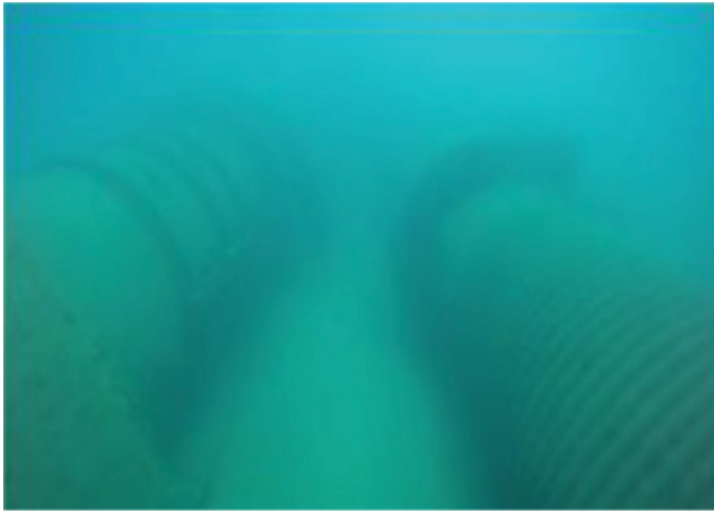
Fig. 6. Seawater catchment pipes from the Tenes desalination plant.
