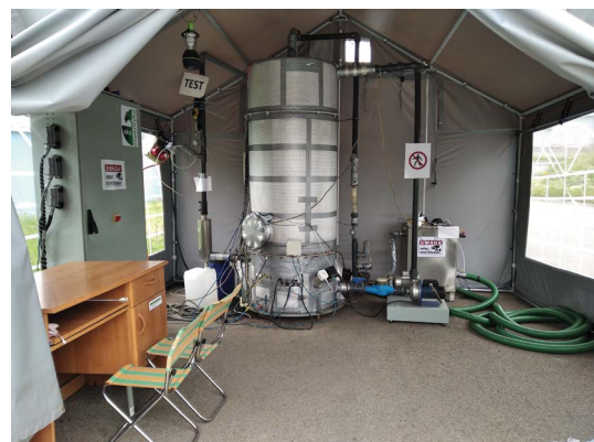
Fig. 1. Pilot-scale compact trickle-bed bioreactor in the wastewater treatment plant.
