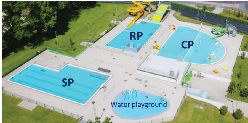
Fig. 1. Tested municipal outdoor swimming pool complex.
