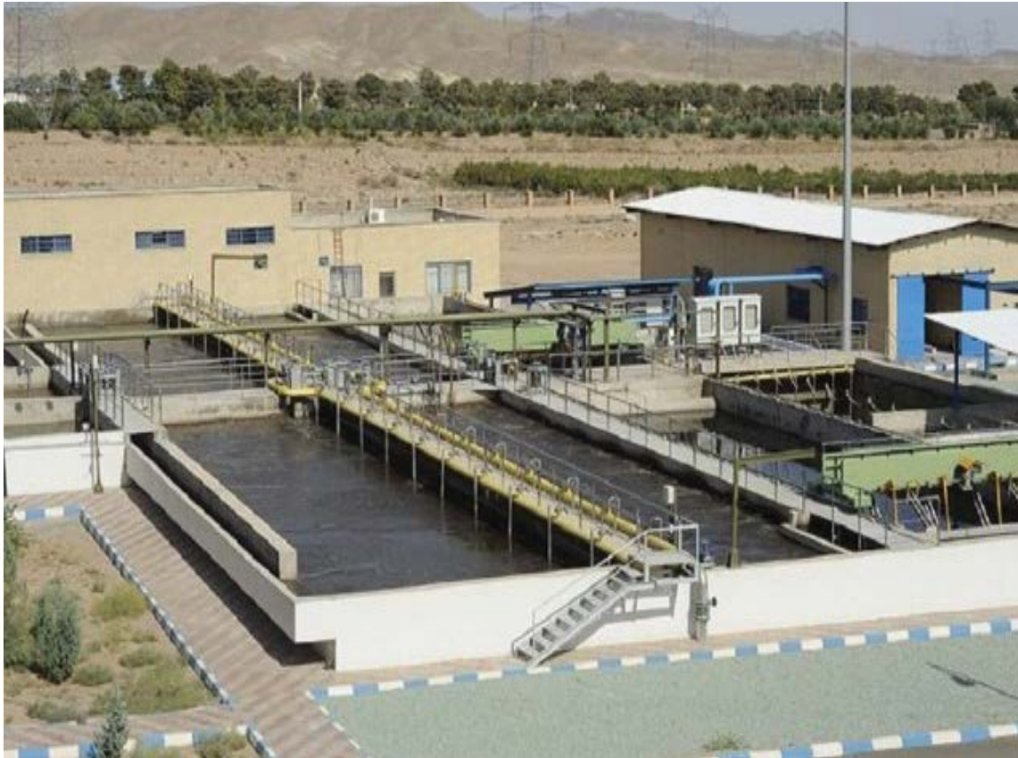
Fig. 1. Ali Ibn Abi Talib hospital wastewater treatment plant in Zahedan City, Iran.
