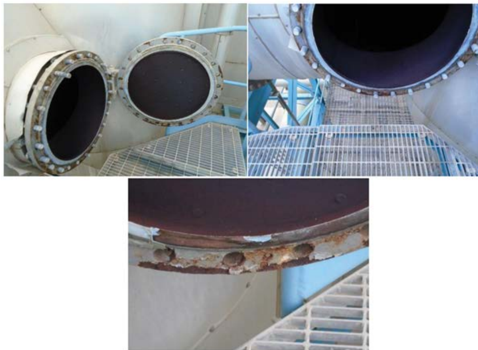
Fig. 15. Unit 23 asbestos gasket removal and protective paint removal.
