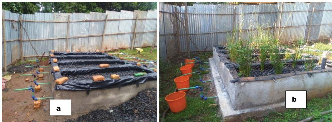
Fig. 4. HSSFCW cells before (a) and after planting with emergent wetland plants (b).
