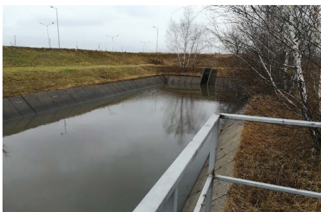
Fig. 1. The catchment area of rainwater from the highway.
