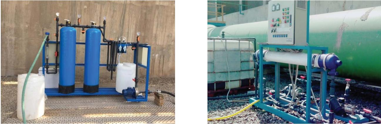
Fig. 4. Media filter (left) and ultrafiltration membrane (right).
