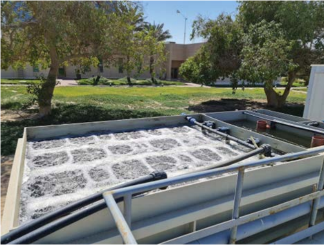
Fig. S1. Side view image of wastewater treatment unit representing (1) aeration tank, (2) secondary settling tanks, and (3) inlet flow stream.
