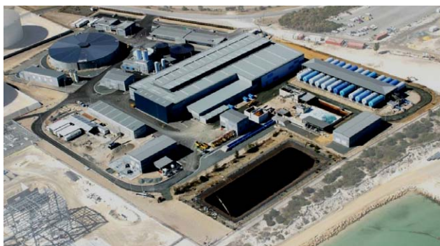
Fig. 8. Perth seawater desalination plant.
