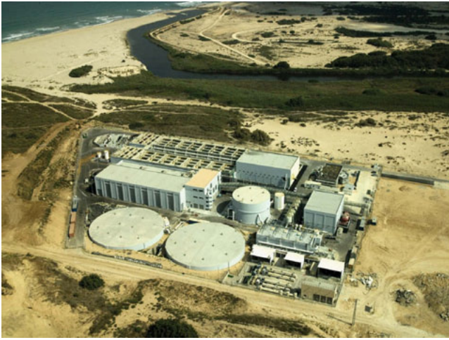
Fig. 1. Palmahim desalination plant general view.
