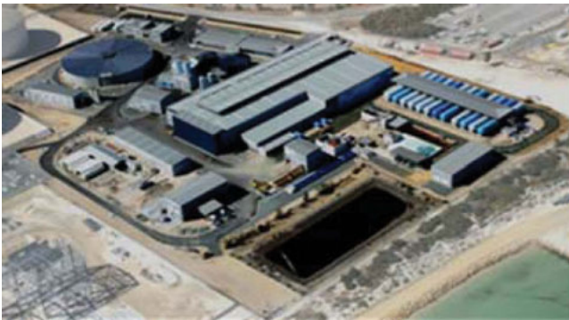
Fig. 1. Perth seawater desalination plant.
