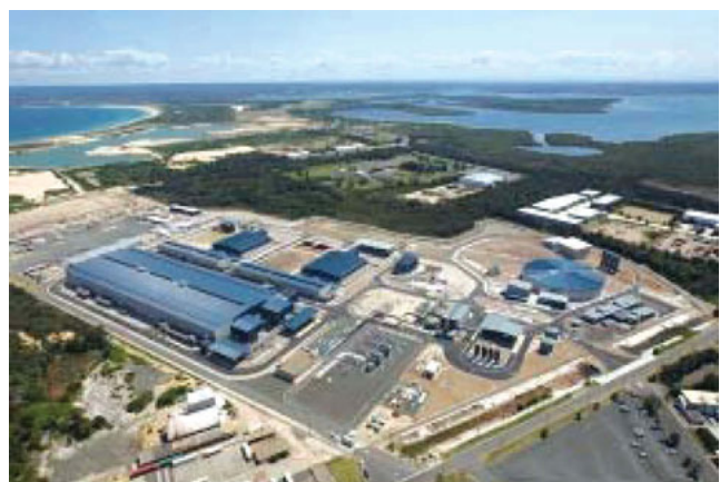
Fig. 4. Sydney desalination plant.
