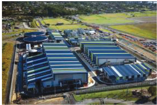
Fig. 3. Gold coast desalination plant.
