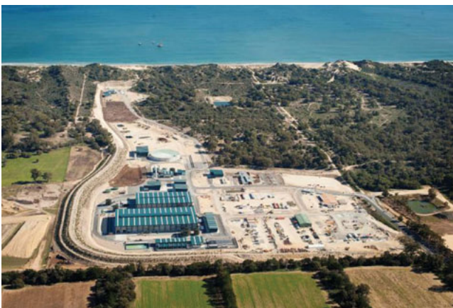
Fig. 2. Southern seawater desalination plant.
