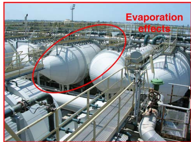
Fig. 3. A picture of evaporation effects of one of the MED-TVC units. Red circle indicates one of the six cylinders containing two subsequent effects.
