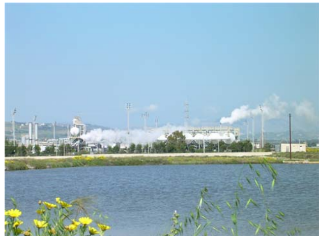
Fig. 4. View of a basin of “Mariastella” saltworks with the MED-TVC plant in the background.
