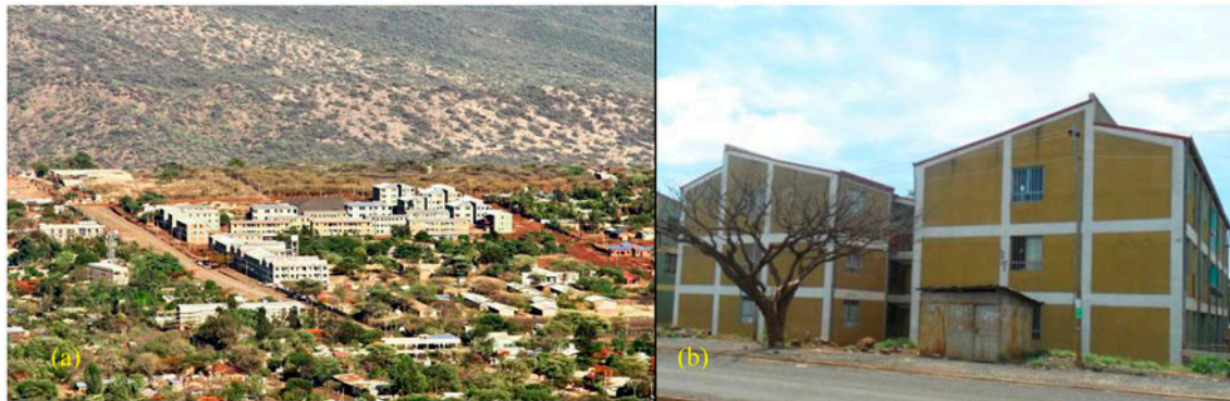
Fig. 1. (a) Bekele Mola condominium houses [7] and (b) two MSBs chosen as pilot plot.
