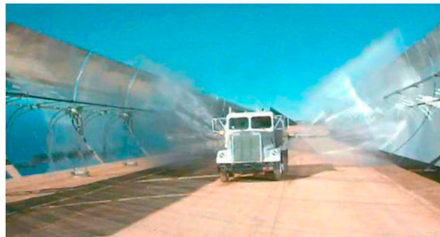
Fig. 20. Trough reflector cleaning at SEGS [23].
