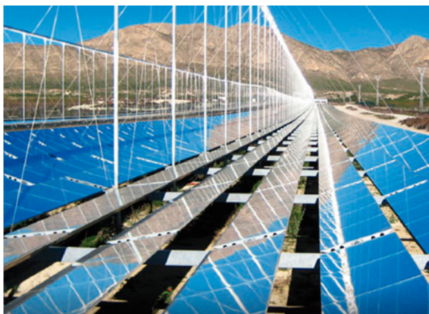
Fig. 13. Fresnel solar collector [13].
