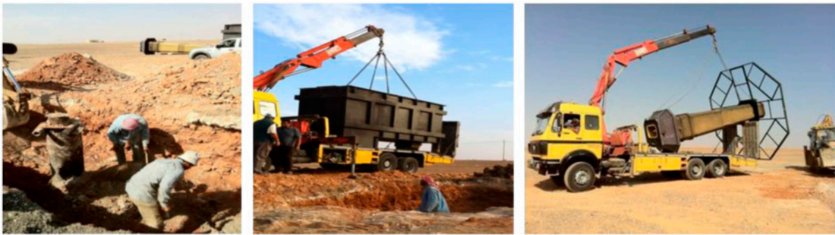
Fig. 11. Indicative photos taken during the installation phase in Jordan.
