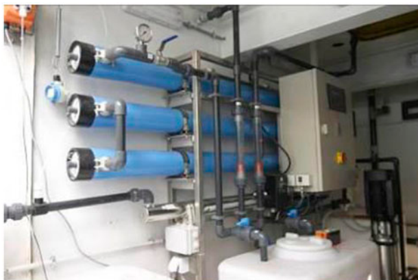
Fig. 5. Indicative view of the RO system including the brackish water pipeline entrance to the main system.
