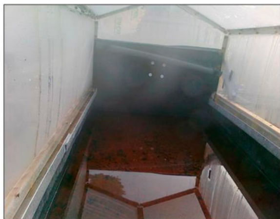
Fig. 6. The shielding surface layer in the control still.
