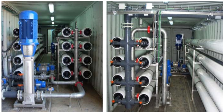
Fig. 2. 835 m 3 /day Reim SWRO-CCD unit.
