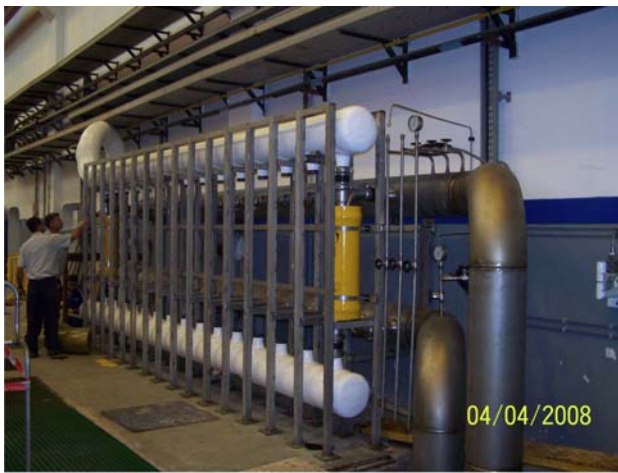
Fig. 9. Installation of the pressure exchangers.
