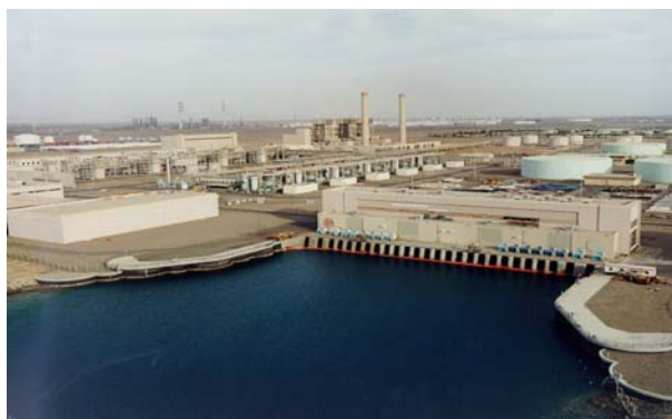
Fig. 1. PD&SC complex with the seawater intake channel in the foreground.
