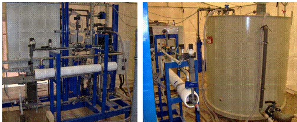
Fig. 2. Photograph of the NF/RO pilot plant (Tan Tan, Morocco, 2008).
