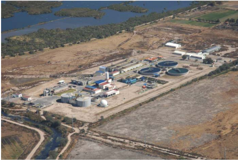
Picture 1. Tenorio municipal waste water treatment plant.
