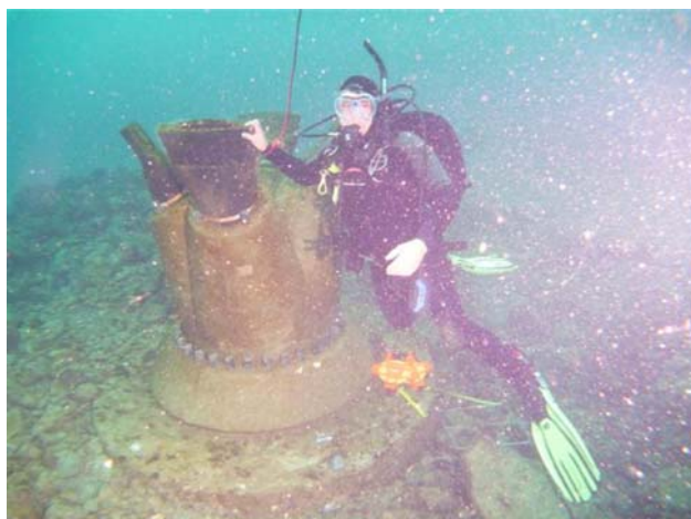
Fig. 3. Photo of diffuser for Adelaide Desalination Plant.
