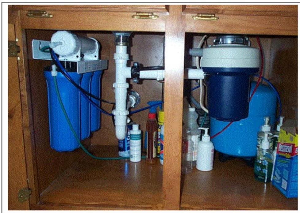
Fig. 2. Photograph showing a RO-based POU water treatment system for the removal of uranium from drinking water (taken with permission from http://www.scdhec.gov/environment/water/urro.htm , South California, Department of health and environmental control) [25].
