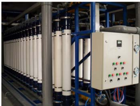
Fig. 3. UF membrane frame actually install figure.
