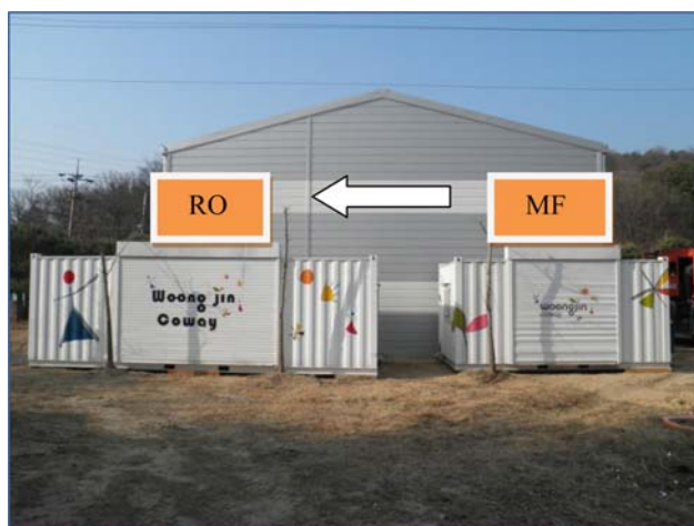
Photo 1. The deployment of MF (30 m 3 /d) and RO (20 m 3 /d) membrane systems of pilot plant.
