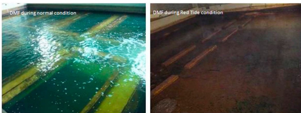
Fig. 2. Thick floating sludge or scum accumulated on top of DMF (right side photograph) during red tide period as compared to clean surface during normal operations (left side photograph) in an operating plant in UAE.
