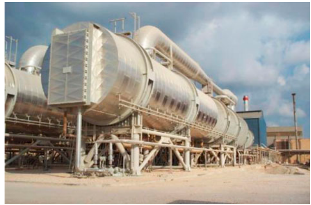
Fig. 24(a). Six effects–13,333 m 3 /d unit with TVC in Tobruk, Libya, in circular vessel along the TC.
