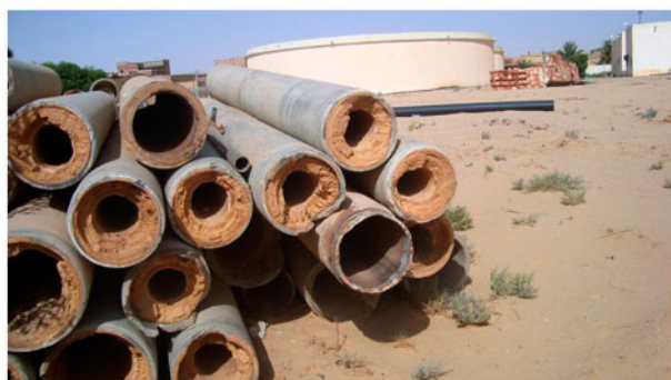
Fig. 5. Renovation of water mains in the Touggourt city (photo 2010).
