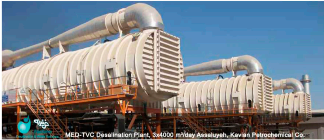
Fig. 3. Experimental MED-TVC units installed in Assalluyeh in Kavian Petrochemical Company [12].
