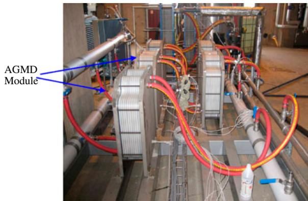
Fig. 17. The five-module Scarab AB system installed at Idbäcken Cogeneration Facility (Nyköping) in Sweden.
