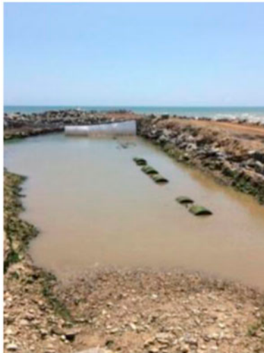
Fig. 13. Site 2—temporary intake.
