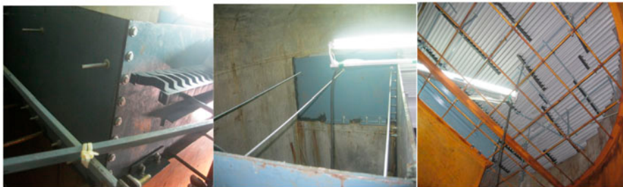
Fig. 13. Demister pad elevation with extended vapor duct.
