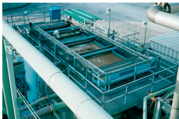
Fig. 7. Horizontal dissolved air flotation system, (DAF) [14].
