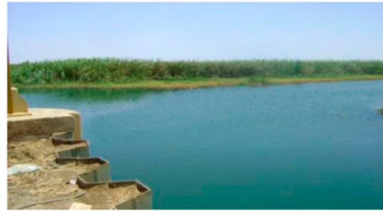
Fig. 3. The water intake from Aftout Es Saheli.
