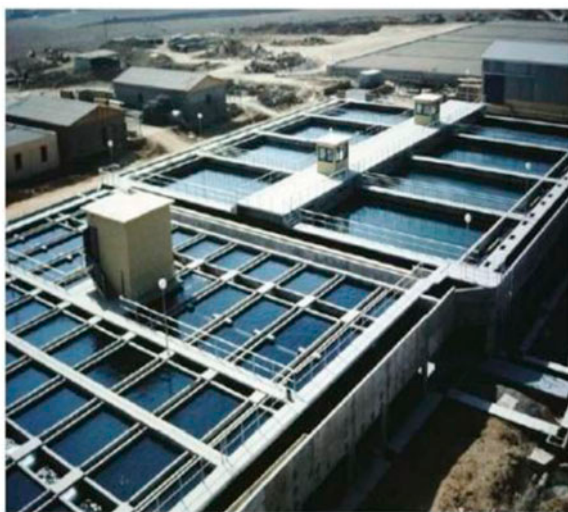
Fig. 5. Pulsa tube clarifier.
