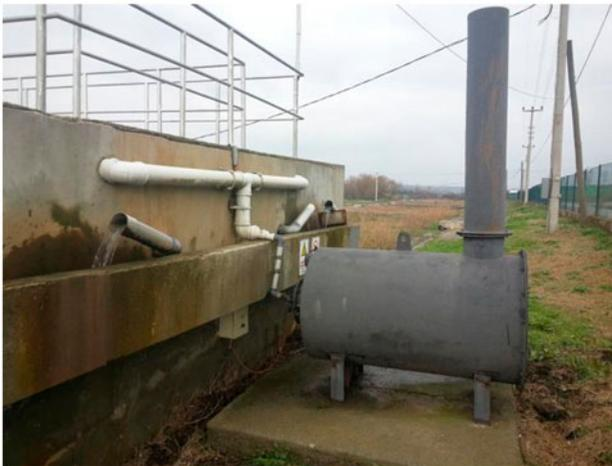
Fig. 2. Gas collection and burning system in anaerobic reactor of Balcik (photo from the system).
