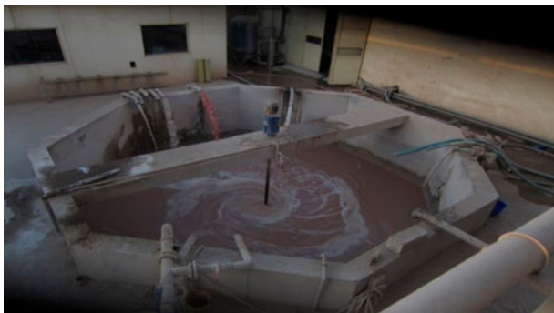
Fig. 1. Equalization tank with different inflows of industrial wastewater.
