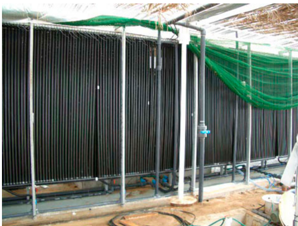
Fig. 1. Photo of the condenser in the seawater greenhouse at Al-Hail, Muscat, Oman.
