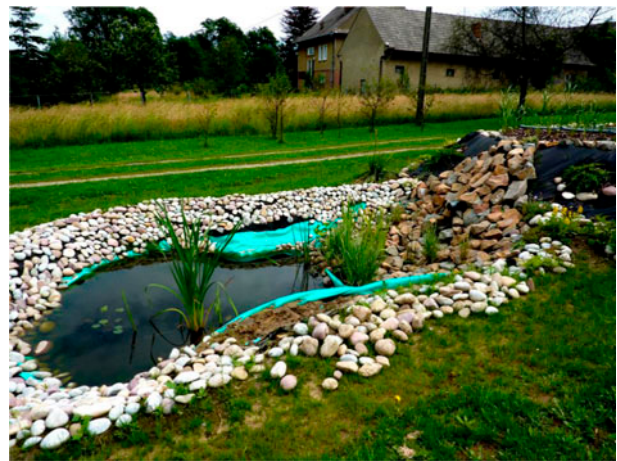
Fig. 4. A view of the effluent polishing pond (photo: author).
