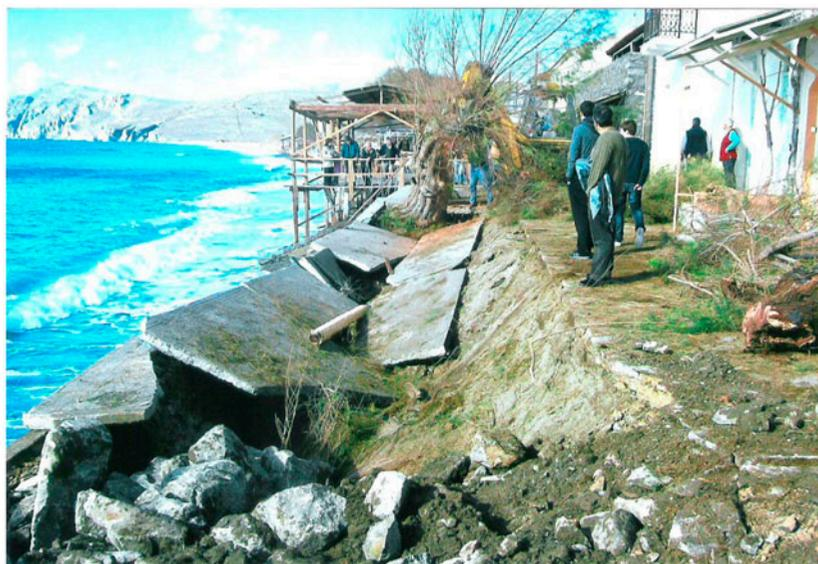
Fig. 7. Sea wall failure due to extreme sea level rise in Eressos coast, Lesbos, Greece.
