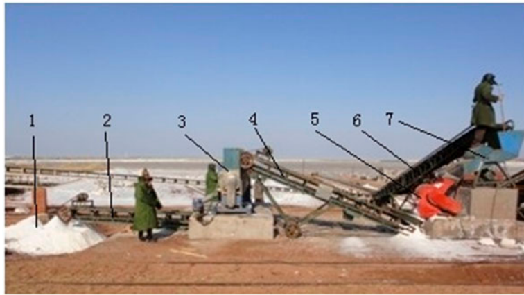
Fig. 8. Continuous desalination equipment (1) production ice; (2) conveyor belt for production ice; (3) centrifuge machine; (4) conveyor belt for ice particles; (5) drum-type ice crusher; (6) hammer crusher; (7) conveyor belt for big block sea ice.
