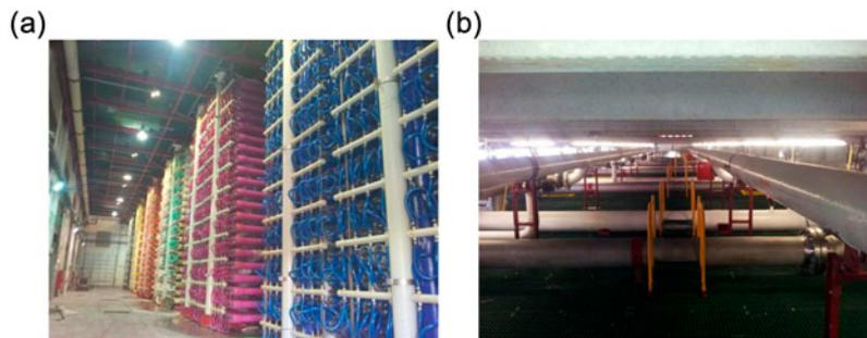
Picture 2. (a) SWRO membrane hall, on the top side of picture the steel beams of the upper platform can be seen. (b) SWRO membrane hall upper platform: HP, LP, and CIP piping.
