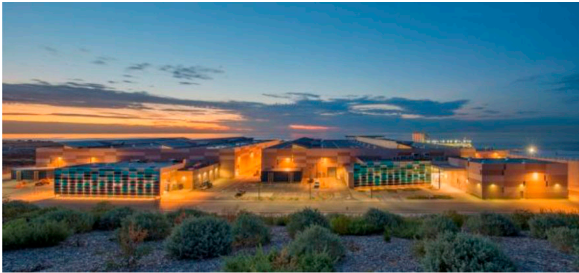
Fig. 1. Adelaide desalination plant.
