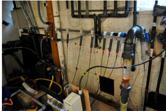
Fig. 3. Schematic drawing and photograph of the 2 m-long monitored superduplex stainless steel pipe.
