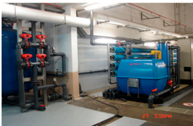
Fig. 10. Pictures of Canary Islands SWRO desalination unit.
